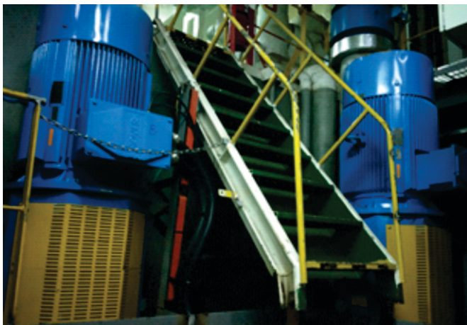
Sea water pump with VFD control
