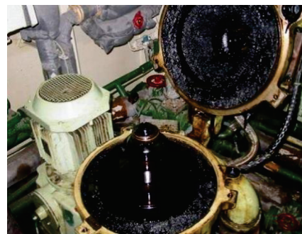
FUEL LINES CHOKED
